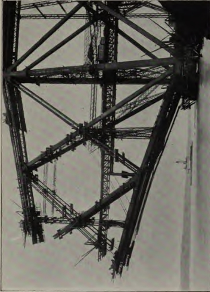
INCH GARVIE MAIN PIER. South Cantilever, Sept. 1888.
